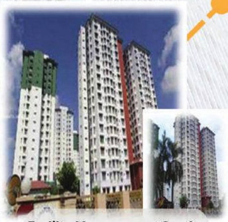
Facility Management Service @ Pangsapuri Ilham, TTDI Jaya, Shah Alam
